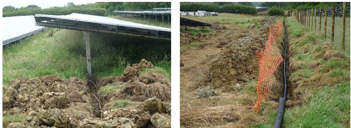
Cabling Channels
